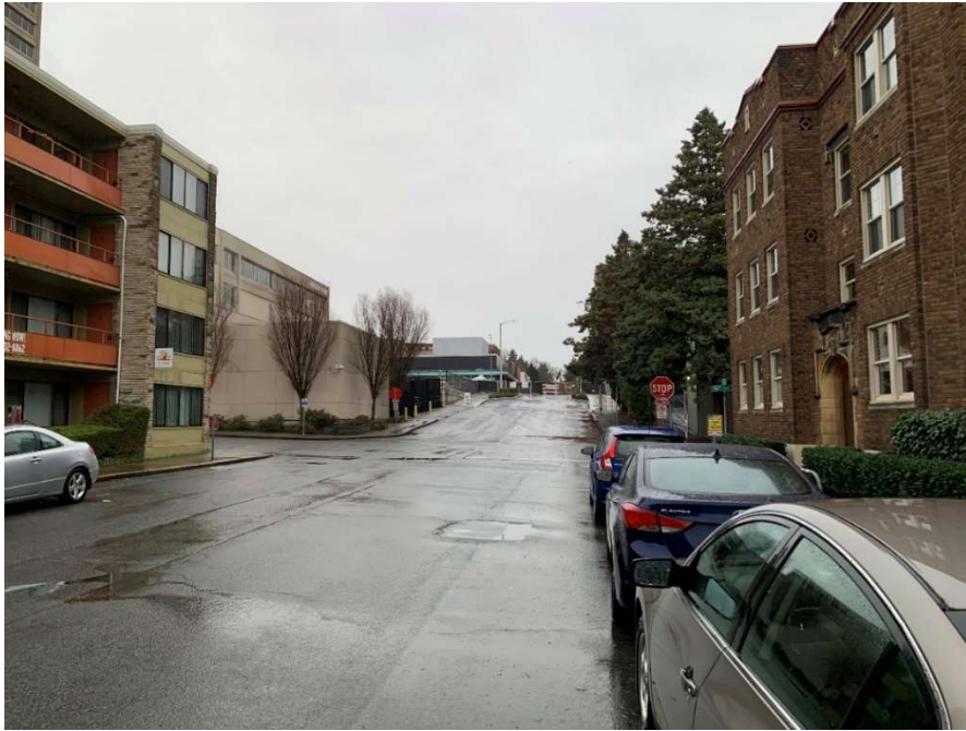
Figure 2-1. Existing Conditions Looking East along NE 43rd St from 11th Ave NE
